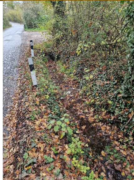
Road ditch to the south of the site.
